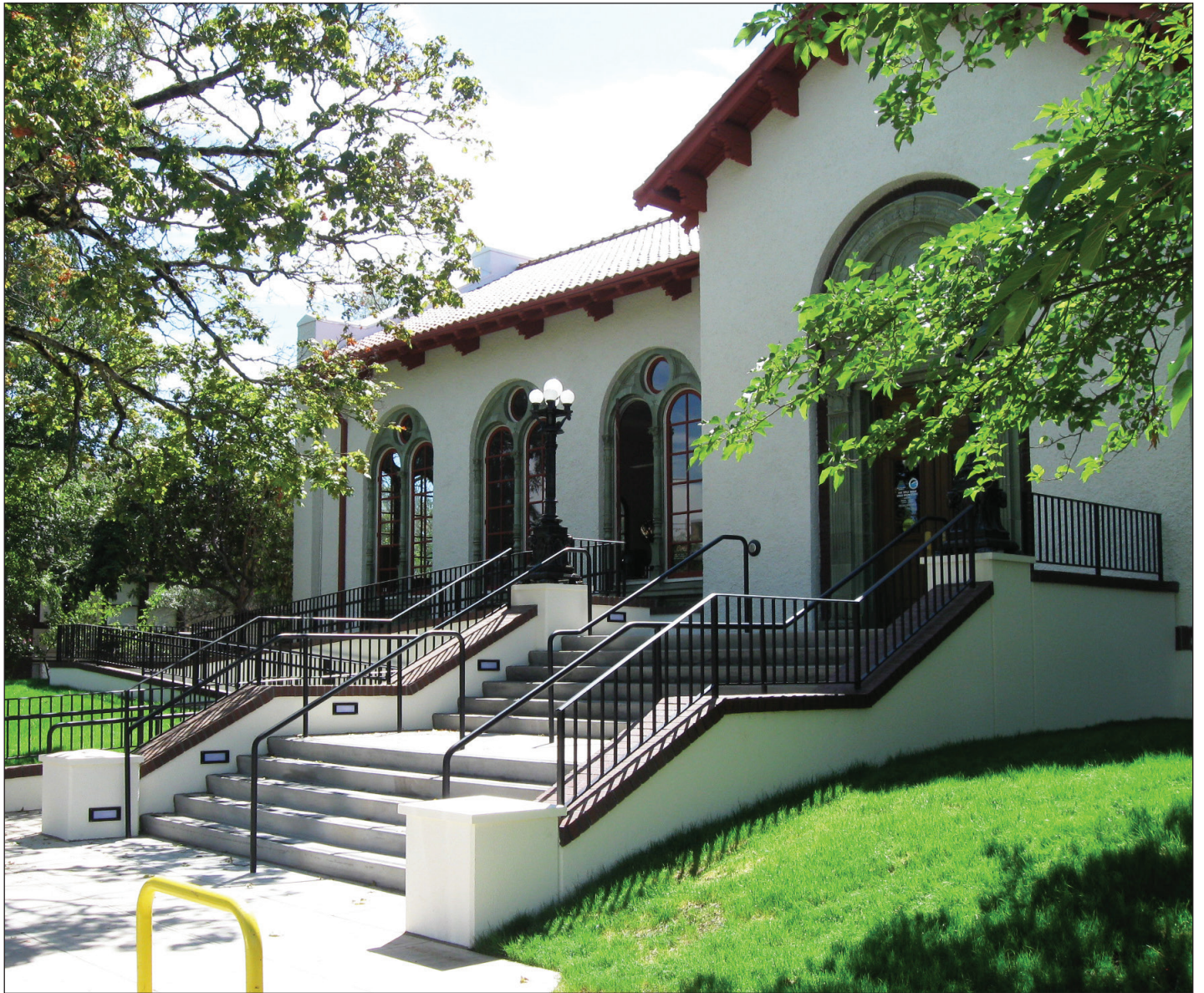
The 1912 Carnegie building, 216 N.E. Knott St., will remain part of an enlarged Albina library that is in the planning stage. Entrance to the new wing will be on Russell Street. (Multnomah County Library)
