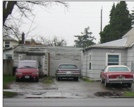
This two-vehicle garage built in 1911 in Arbor Lodge along North Rosa Parks Way is slated to be removed by the owners of adjoining properties. (BDS)
