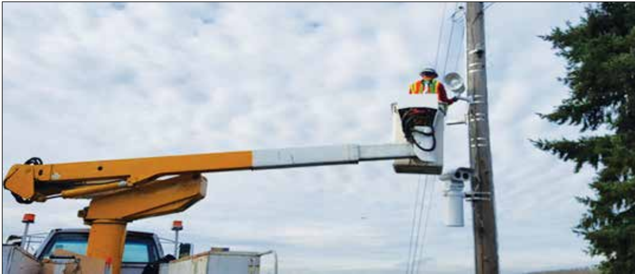
A Portland Transportation Bureau contractor installs a speed camera on a high-crash corridor. The bureau will double the number of cameras this year and next on Portland's most dangerous streets and intersections. (PBOT)
