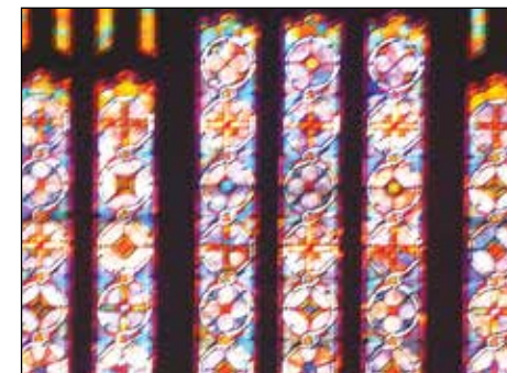
A plastic covering has been removed from the window on the north side of Westminster Presbyterian Church. A laminated glass, like a car windshield, with a ventilating feature now protects the stained glass. (Janet Goetze)
