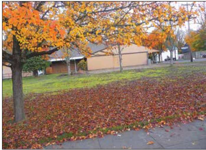
Portsmouth United Church demolished one wing to clear its side yard at Fiske Avenue and Lombard Street. Members will spend the winter completing paper work for zoning and permits, with construction of 20 affordable housing units expected next spring. Other churches are starting to look at ways to ease Portland's housing shortage. (Janet Goetze)
