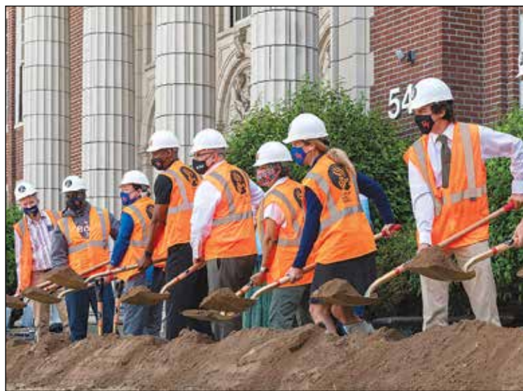
A ground breaking ceremony was held in August for the three-year modernization project of Benson Polytechnic High School, at 546 N.E. 12th Ave. in the Kerns neighborhood. City permits have been approved for demolition of attached buildings and sections of the main building where additions are planned. (Portland Public Schools)
