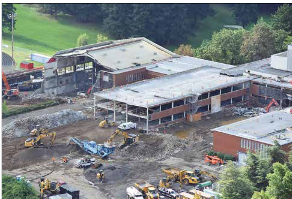
Demolition work has begun on the Madison High School modernization project.. (Portland Public Schools)
