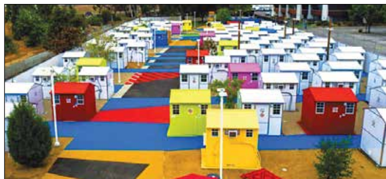
In a move to replace tent cities with small structures, officials envision Safe Rest Villages in as many as 70 sites around the city. Most potential sites are in North Portland. (City of Portland)
