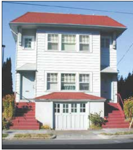
A Seattle-based trust, owner of this Lloyd District fire-damaged duplex built in 1911, is seeking permission to deconstruct the building, claiming it is a dangerous structure. (Portland Bureau of Environmental Services)
