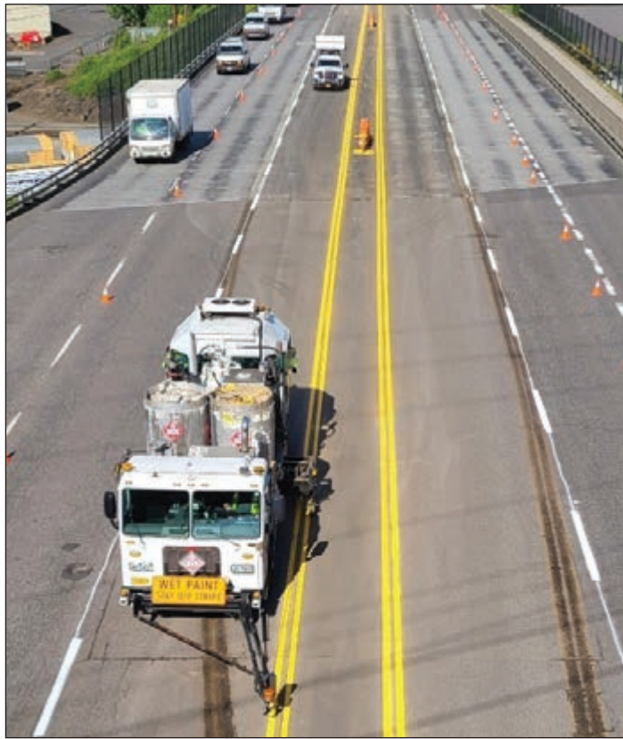
Portland Bureau of Transportation crews finish line striping on the North Going Street Bridge lanes. A multiyear project restored the span's six traffic lanes for access to Swan Island, a key industrial area for the region. (PBOT)
