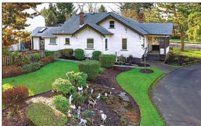
In a single day, what was once a well-maintained property at 5506 N.E. Simpson St. became a leveled lot waiting for future development. Cully neighbors have referred the quick demolition to the Multnomah County District Attorney's office for possible criminal prosecution over inadequate lead testing. (Zillow)
