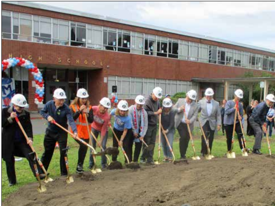
Public officials, students, neighbors and former Rose Festival princesses helped break ground in mid-May for the renovation of Madison High School in Northeast Portland. Work is expected to be completed in August 2021. (Phill Colombo)
