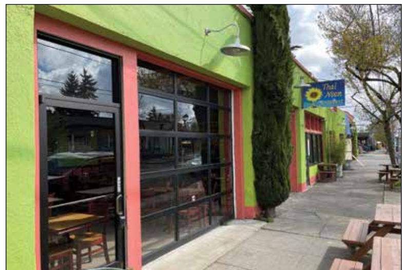
A Concordia commercial building built in 1917 at 2630-2640 N.E. Alberta St. is undergoing upfitting of its 4,000-square-foot space. Owner Melissa Jackson is adding a new tenant to a long-unused space. (Phill Colombo)
