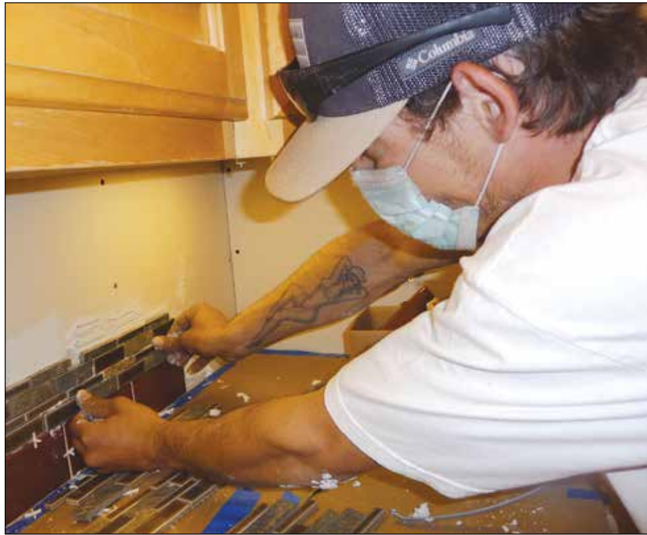
Andrew Linn sets tile for a kitchen backsplash by pressing the tile into place. (Janet Goetze)
