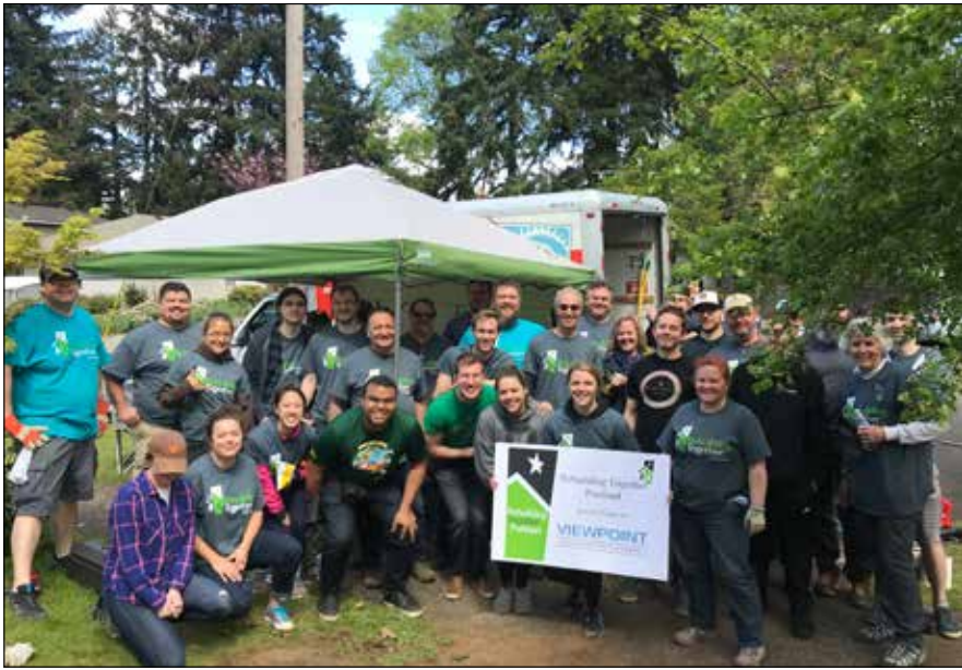
A volunteer crew from Viewpoint, a local software construction firm, give up their Saturday to rehabilitate a Madison South property for an elderly homeowner. (Dana Busch)
