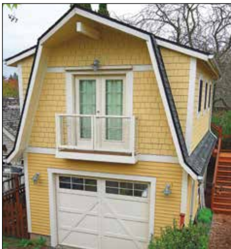
Miles TeSelle and Holly Hood converted a garage to include a second-story ADU as a rental in the Roseway neighborhood. The ADU replicates the farmhouse architectural style of the primary house, complete with gambrel dormers. (John Butenschoen)
