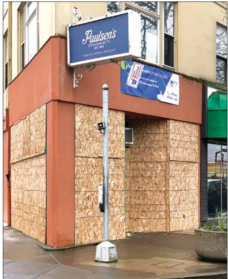
Paulsen's Pharmacy closed in January and is likely to stay vacant until at least April, when its lease expires. During recent storm conditions, Joe Amspoker boarded the windows and doors after three break-in alarms. "People basically broke into the front door," he said. "I think they were looking for a warm place." (Nancy Varekamp)
