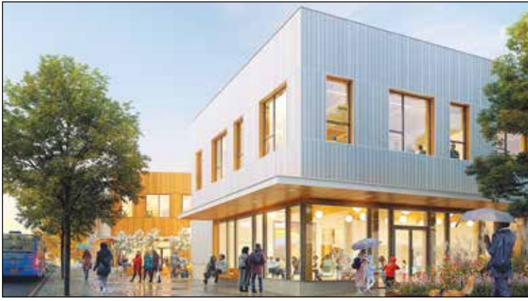
Ground was broken in late January for construction of 84 affordable housing units at PCC's Metropolitan Workforce center in Cully. The new units will allow students to live where they train to gain employment skills. Home Forward has partnered with PCC to develop, build and operate the project. (Bora Architects)
