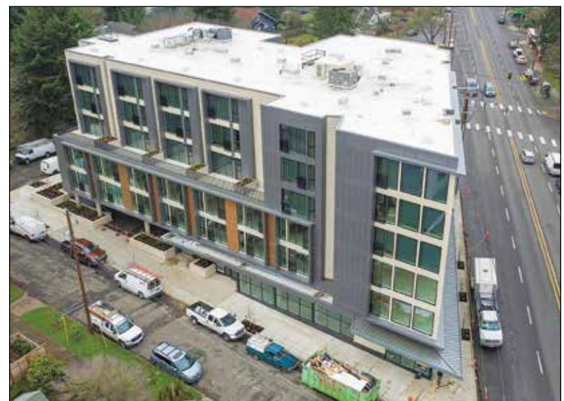
Set for occupancy by mid-February, Sandy 51 began leasing in January. The six-story, 86-unit building will have 4000 square feet of commercial space and 19 parking spaces on the ground floor. (Stratoscope)
