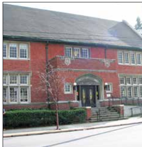
North Portland Library in Humboldt is one of several that will close for renovation and expansion in the spring of 2023. (Multnomah County Library)
