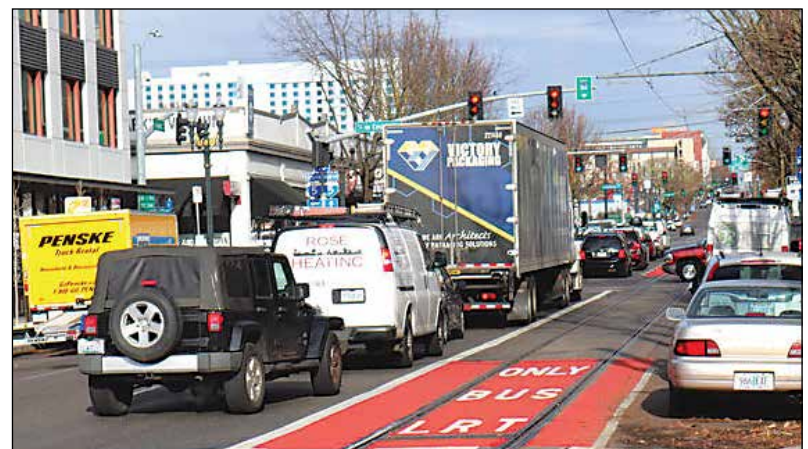
A previously installed Rose Lane on Northeast Grand Avenue between Burnside and Couch Streets. (Pierre Haou, Portland Bureau of Transportation)
